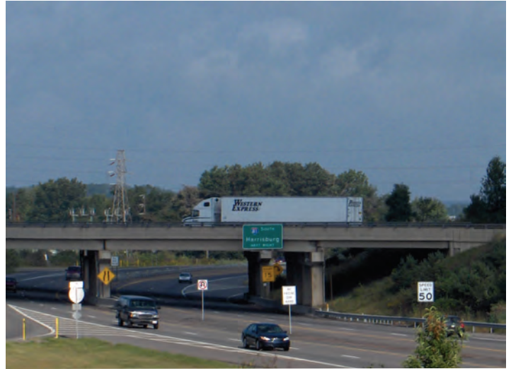
Interstate 81 poses the largest potential threat to most of the systems involved in the Upper Schuylkill Watershed effort.
